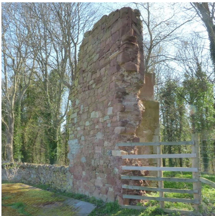
Figure 4. The remains of Papple Hall. A window embrasure can be seen at the top facing with the c1855 water-supply tanks behind.
