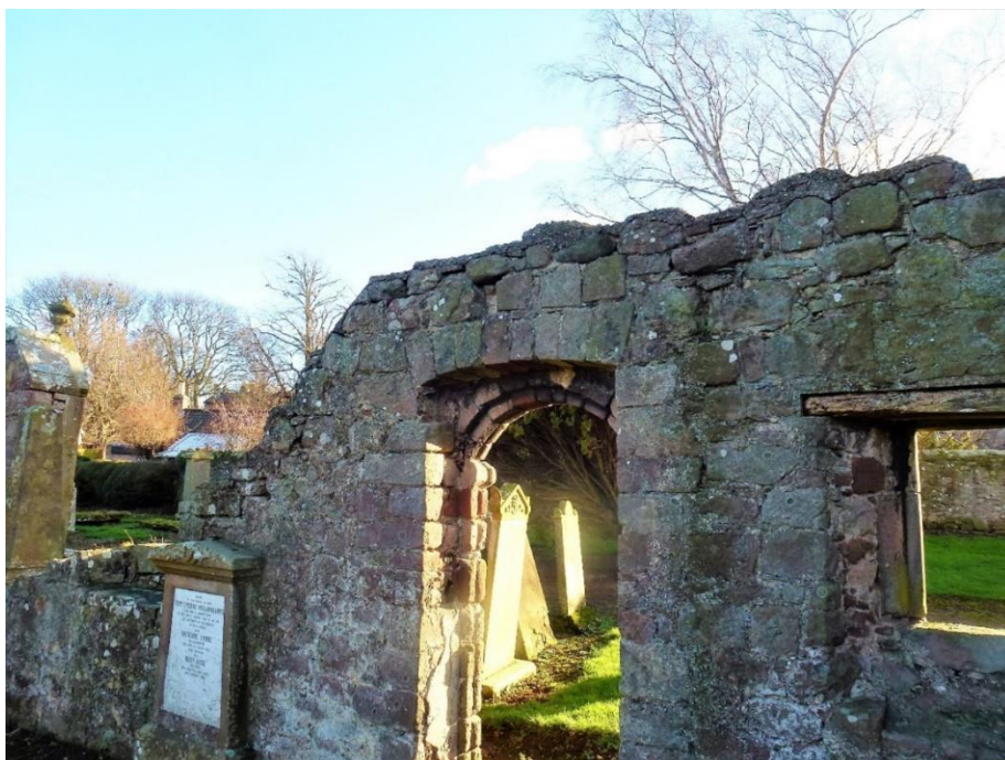
Figure 2. Stenton Church. Back of the doorway and, to its right, under-loft window, showing their different construction.
