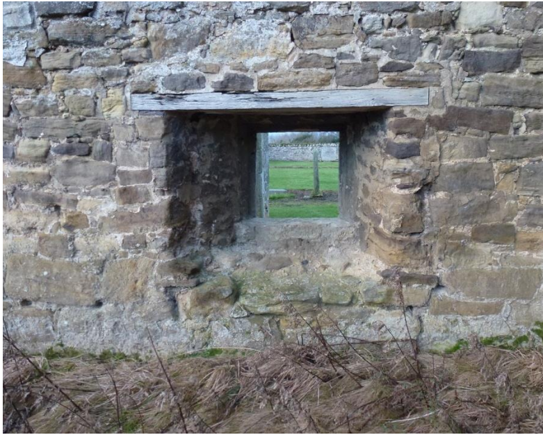
Figure 5. Gladsmuir Kirk. The interior of the south-west window, with wooden lintel.
