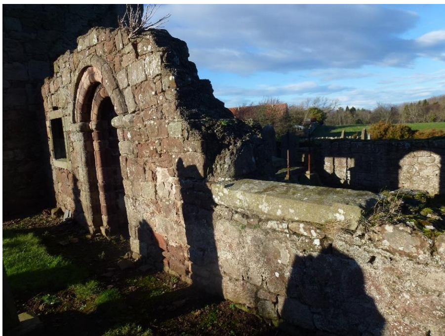
Figure 3. Stenton Church. South wall showing large window inserted into the nave.
