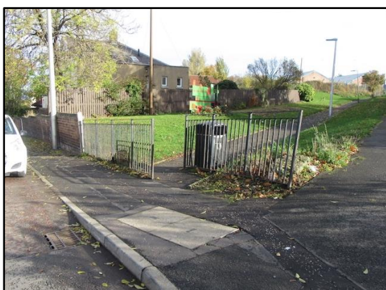
Culvert on Salters Road
