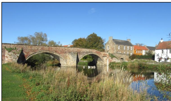
Nungate Bridge, Haddington
