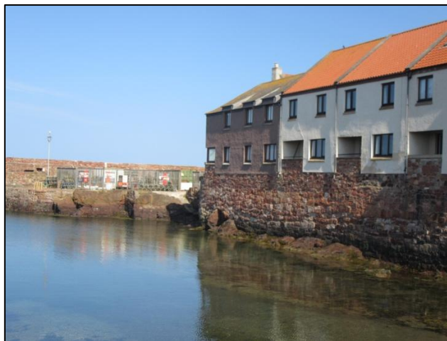
Broad Haven, Dunbar: probable site of the 'loading rock'
