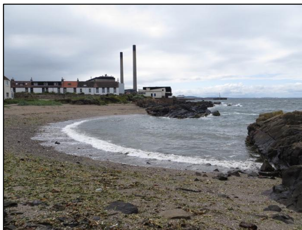
Cockenzie, the Boatshore, before demolition of the power station
