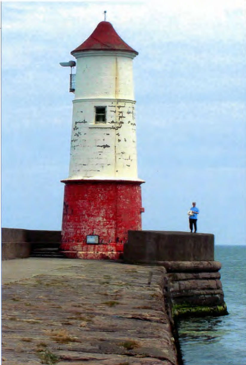
Rennie's Berwick Pier and lighthouse 1808-24. About 30 ft Wide and 2000 ft long cost £63,000 – still in service
