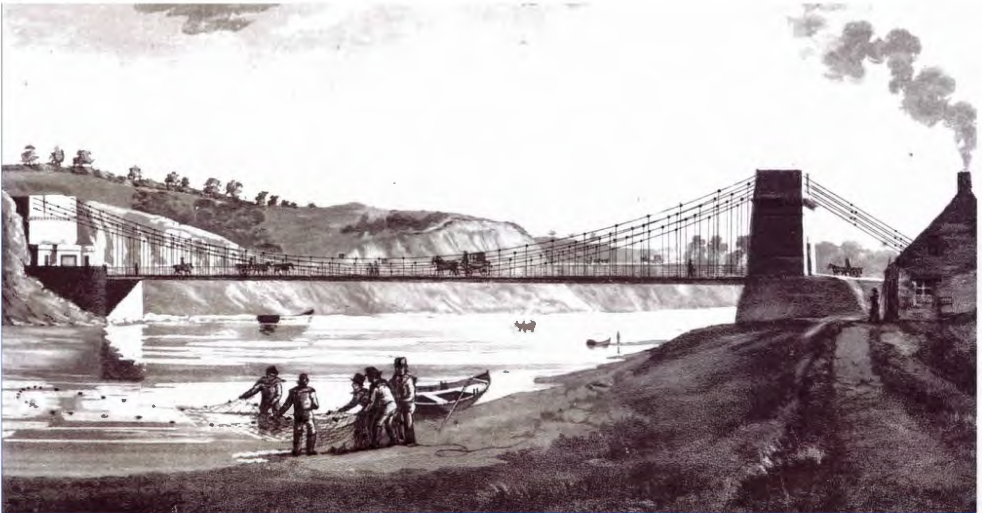
Union Bridge, Paxton 1819-20. Rennie advised on the strengthening of the tower and abutment. Capt. Brown, Engineer The world's oldest suspension bridge still carrying vehicles
