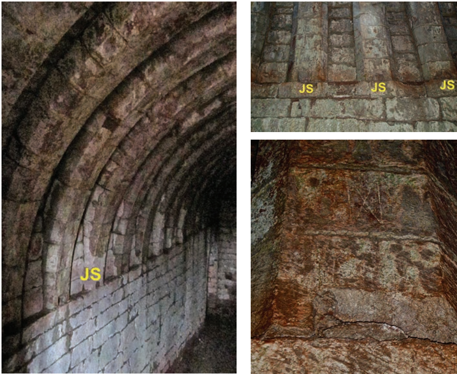
Figure 14: (left) The finely-constructed vault ribs along the west side (Dec 2013), and (top right) some of the joist sockets (JS) crudely cut into the side walls to carry an inserted upper floor (March 2014). (Bottom right) A joist socket (JS) cut through an original mason's mark (April 2016).
