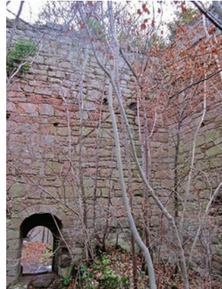
Figure 8: The inner face of the north curtain wall (east end) showing the roof-raggle of a demolished building (Dec 2013).
