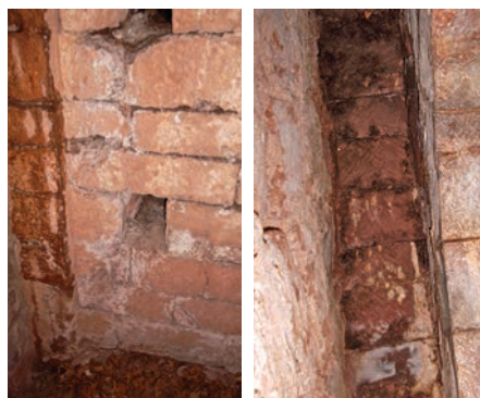
Figure 16: (left) The two draw-bar slots at the west doorway, and (right) the portcullis (?) slot behind that door (April 2016).
