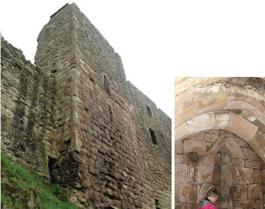
Figure 19: (Left) the tower-keep at Hailes Castle, built contemporaneously with the Goblin Ha', and (right) the fine pointed vault in its basement prison. (Photos: Chris Tabraham)
