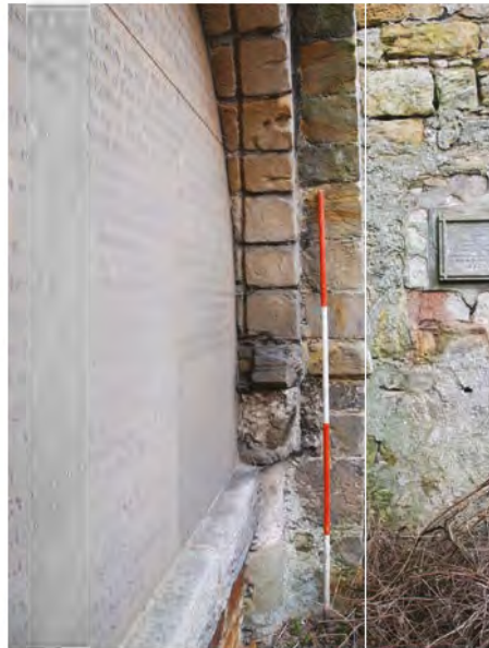
Figure 13: Detail of the groove on the soffit of the chancel arch.
