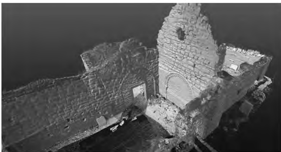
Figure 10: 'Point cloud' data from the scan of the kirk, from the south-west showing the chancel arch.
