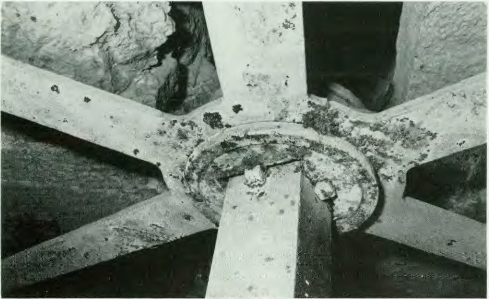
Plate 2. Preston Mill, detail of inside face of water wheel hub and shaft showing split hub and shrink-ring.
